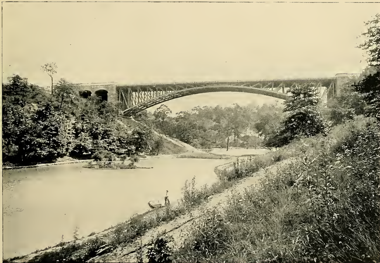
Bridge over Panther Hollow, Schenley Park.
